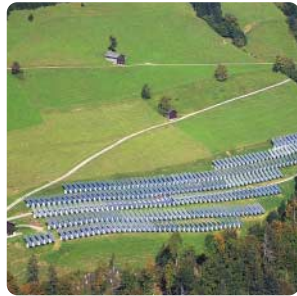
Small power plant
