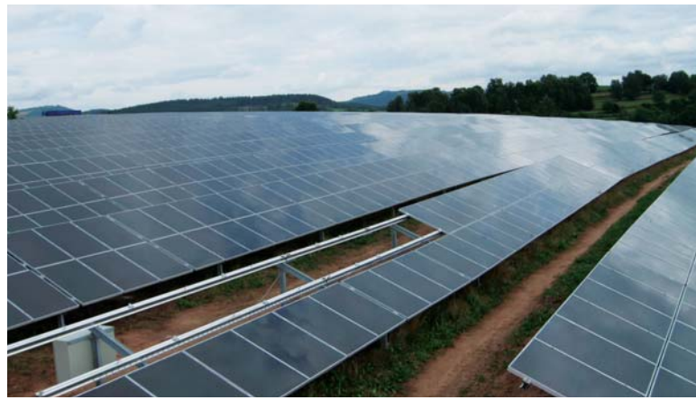
14,100 Sharp amorphous silicon thin film modules power a 1.63 MW array in Viernau, Germany.
