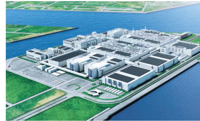
MANUFACTURING COMPLEX FOR THE 21ST CENTURY: SAKAI CITY FACTORY. With a projected production capacity of one gigawatt, Sharp's new, state-of-the-art industrial complex is scheduled to begin producing thin film solar in 2010. The largest factory of its kind, the Sakai plant will also produce its own electricity with an 18-megawatt roof-mounted solar system.
