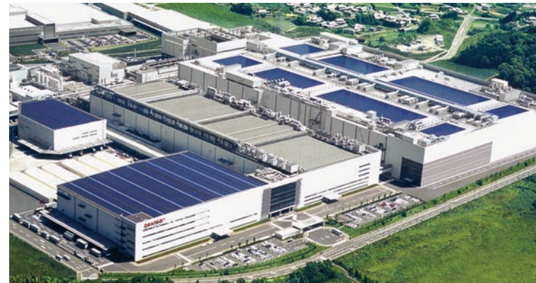
A production facility befitting an environmentally-advanced company, the Kameyama LCD Plant features one of the world's largest roof-mounted solar systems, creating enough electricity to power approximately 1,300 homes.
